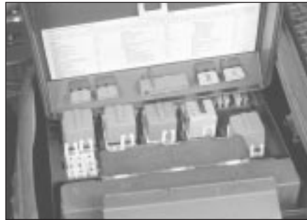
3.1 The fusebox is located in the engine compartment under a cover - the box also includes several relays
